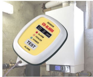
CO Gas Alarm
